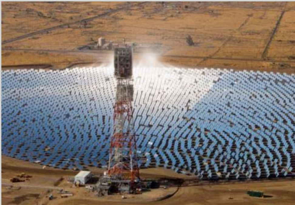
Two flat glass mirrors (2.3m x 3.3m) mounted on a single pylon equipped with a computer-controlled drive system
